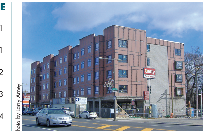
Photo by Larry Arney The finishing touches are being put on our new residence at 2415 N. Broad Street, scheduled to open this summer.
